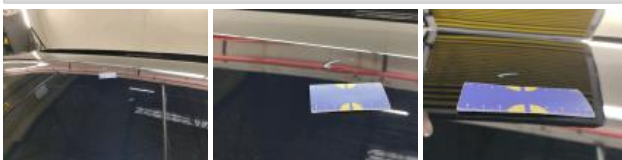
Roof, Dent(s), Acceptable
