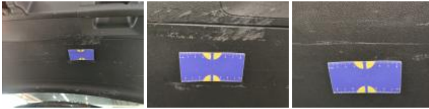
Internal boot lining L, Broken, Smart repair
