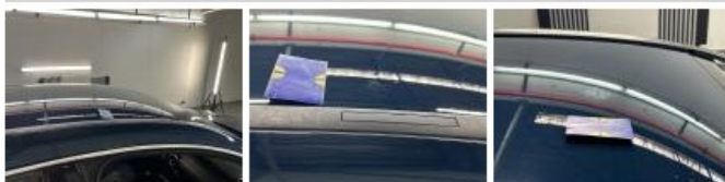
Roof, Chemical polution, Polish
